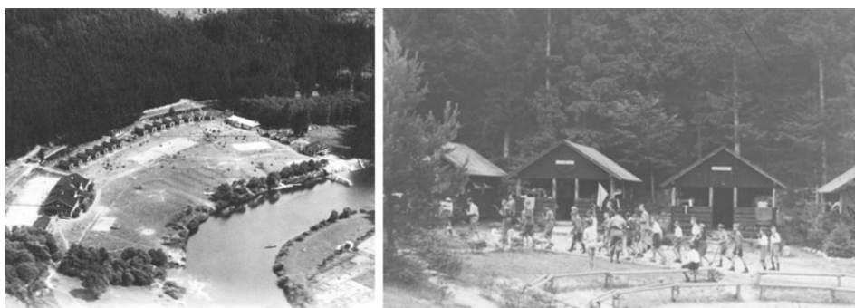
Figure 6. View of the Masaryk Camp on the River Sázava and the Beskid Camp outside the town of Mszana Dolna 84
