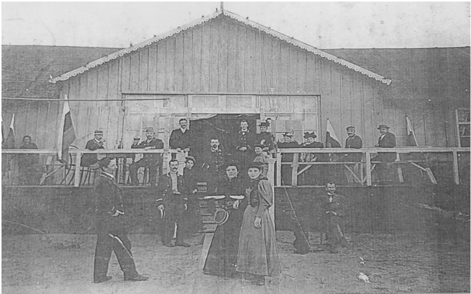
Figure 5. Summer pavilion of the Kamianske Yacht Club (1913)
