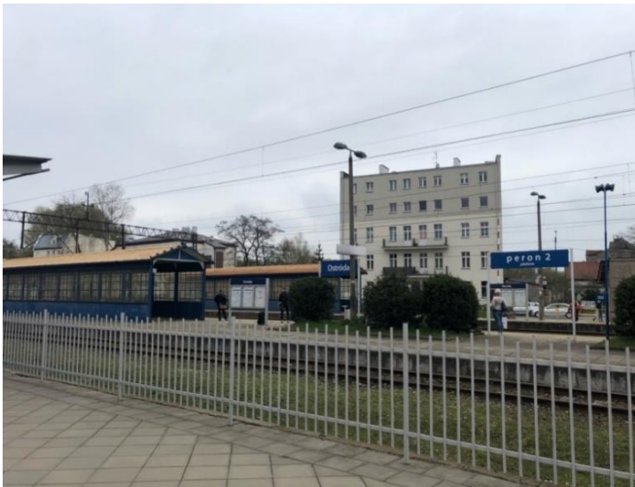
Fig. 2. Railway platform in Ostróda
