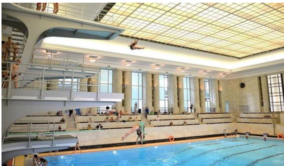
Fig. 5. The Palace of Youth in Warsaw, the indoor swimming pool after modernisation and renovation works in 2016 (source: fotopolska.eu)
