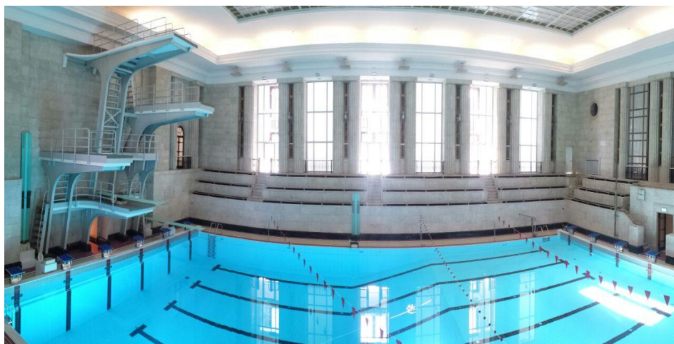
Fig. 4. The Palace of Youth in Warsaw, the indoor swimming pool after modernisation and renovation works in 2016 (source: Bartłomiej Krynicki, 2016)
