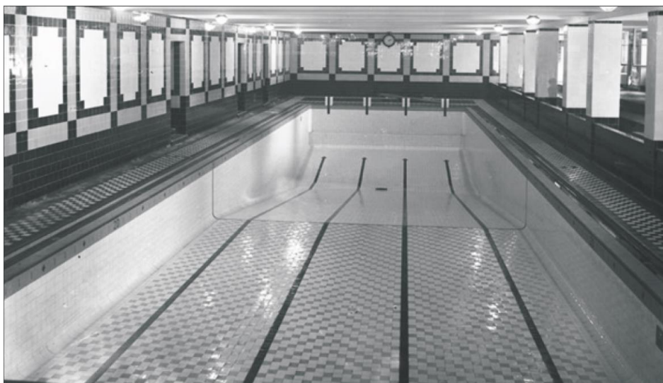
Image 1. Swimming pool YMCA in Kraków, Poland (1927)
