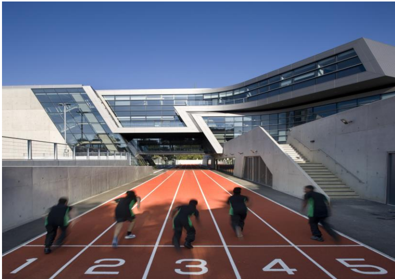
Fig. 6. The newly built secondary school in London (years of construction: 2006–2010). The long track and field track is embracing and ‘encircling’ the school complex, running both outside and inside school buildings (similar to the ancient ‘dromos’ in gymnasiums – allows students to exercise in various weather conditions). Source: www.zaha-hadid.com (access: in July 2016), published with permission obtained from Zaha-Hadid Architects, London.
