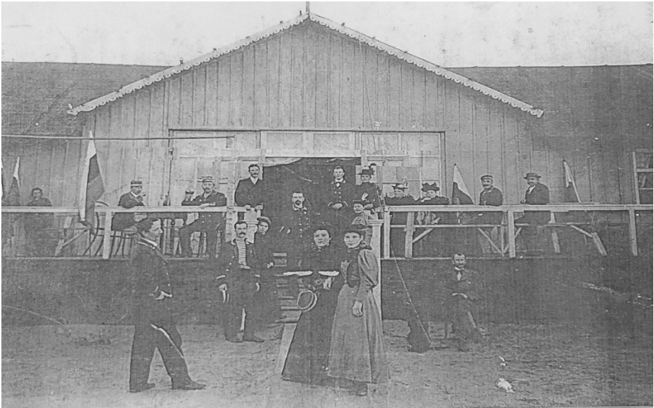
Figure 5. Summer pavilion of the Kamianske Yacht Club (1913)
